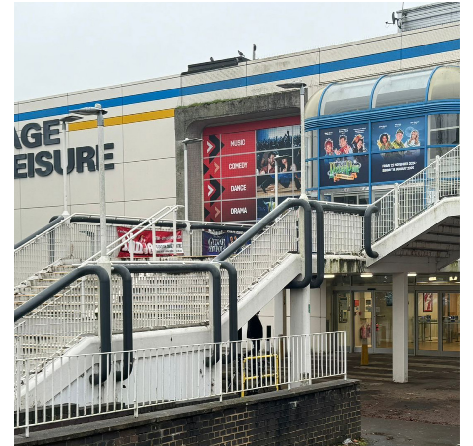
Existing Stevenage Arts & Leisure Centre
