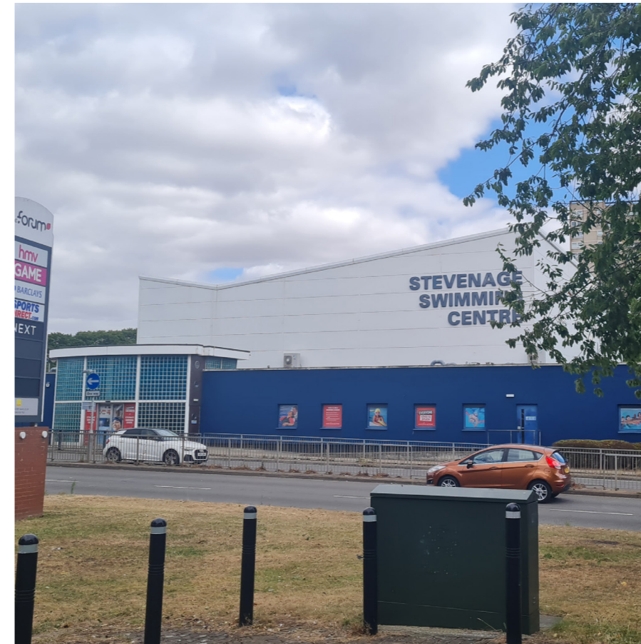
Existing Stevenage Swim Centre
